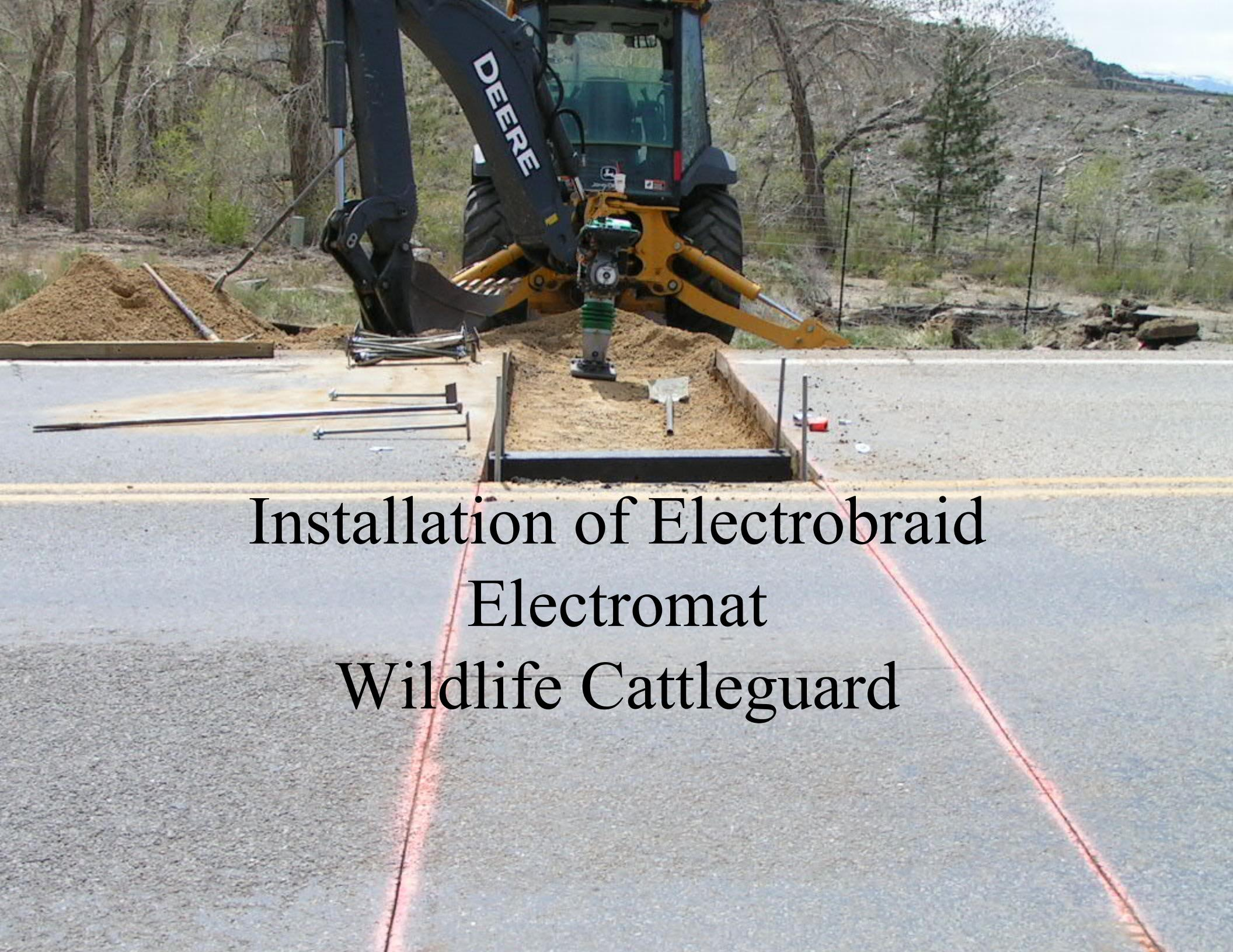
A Deere backhoe loader is shown from a rear three-quarter angle, its arm extended to install a rectangular metal frame into a shallow, rectangular hole it has dug into the ground. The machine is positioned on a paved road. In the background, there's a dirt embankment with sparse vegetation and a fence line. The sky is clear and blue. Red surveying lines are visible on the asphalt road surface.
