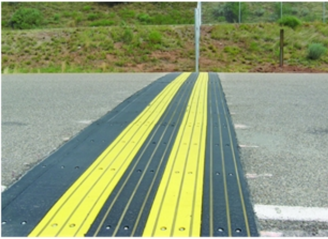
Electromat© at on-ramp in New Mexico
